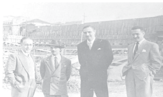
Figure 2 – Launching of the fundamental stone of Cancer Hospital. From left to right, engineer Rino Levi, Mr. Mafra and Professor Prudente
